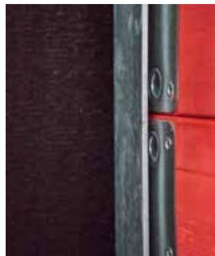
The decks or panels are inserted into the I girder from above, where they then form a stable wall of up to 5 cm in thickness.
