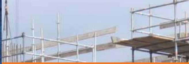
Simplicity, reliability, convenience and efficiency are the foundations of the sturdy RINGSCAFF concept. The optimum combination of a limited number of components creates a stable scaffold structure.
